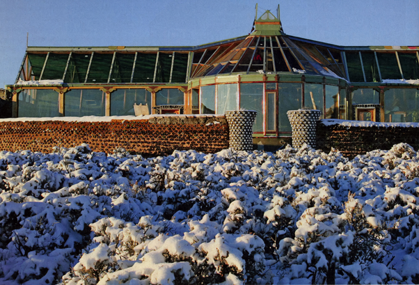
Clockwise from above: Colored panels atop the Phoenix Earthship, near Taos, New Mexico, are made from discarded appliances; a bedroom has a wall fashioned from mud and bottles; a view from the two-story greenhouse; a close-up of a bottle wall.
